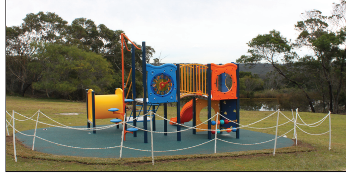
A NEW PLAYGROUND: Through the tireless efforts of the Parents' Committee and donors new playground equipment built to modern standards is installed for primary students in 2014. The college has recently added a computer room.
